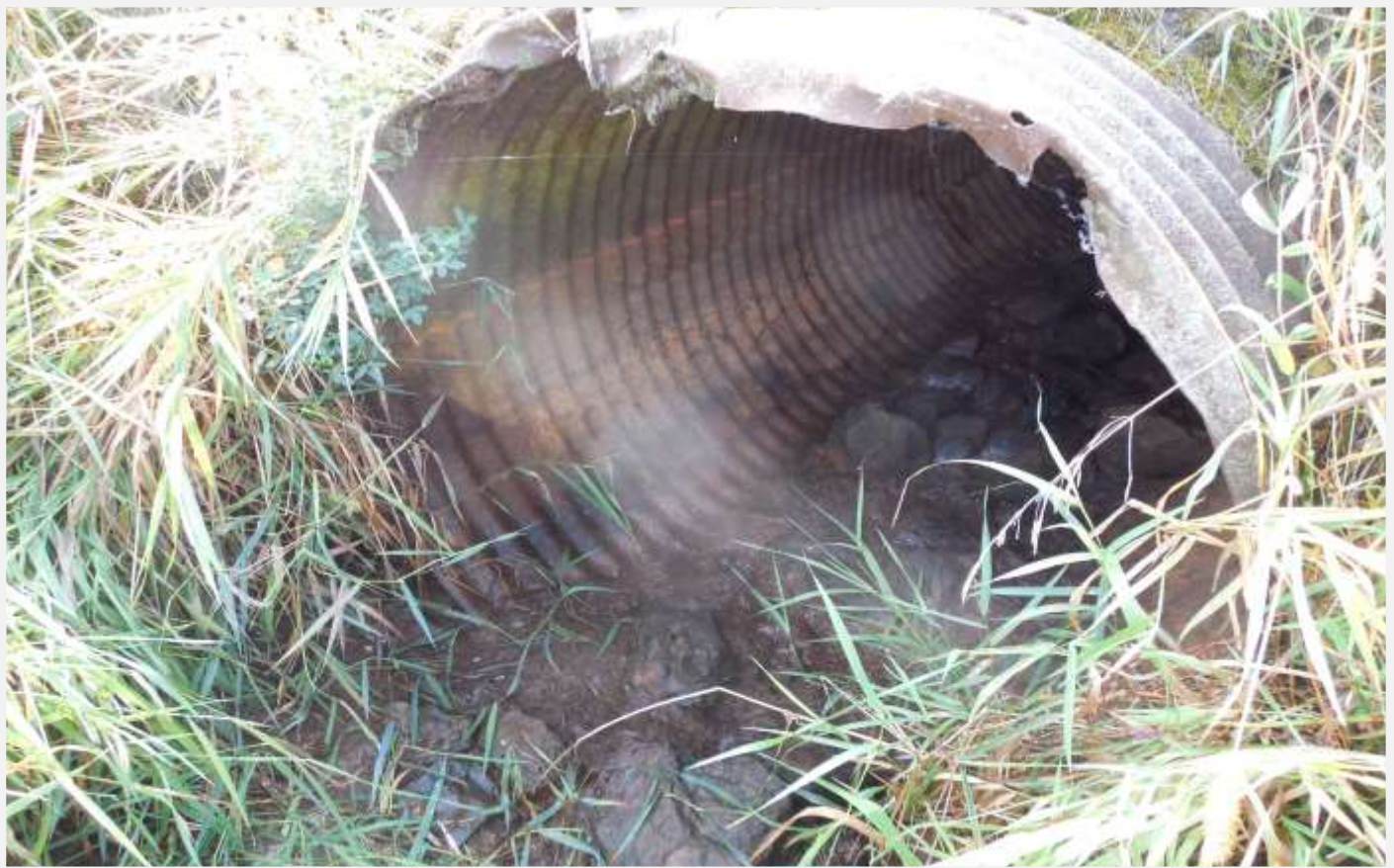
Culvert to be replaced on Isle Avenue.
