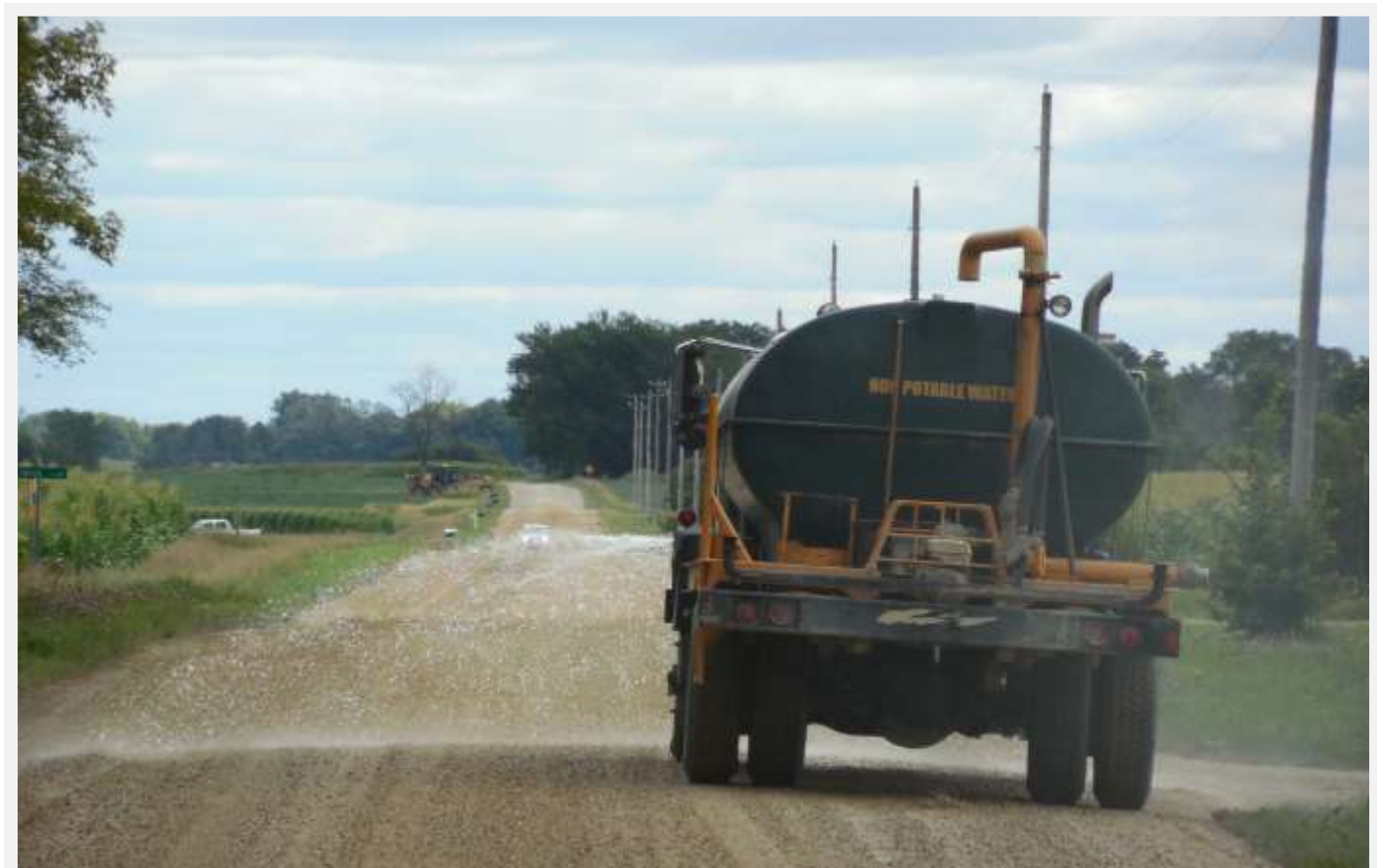
Water application during grading of new aggregate.
