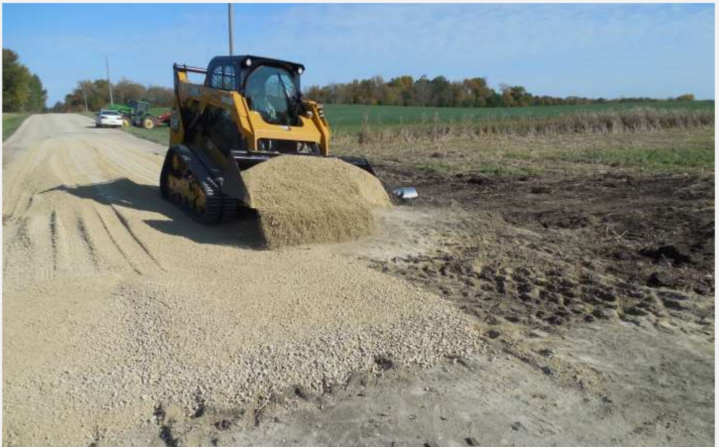
Finishing the Isle Avenue road surface.
