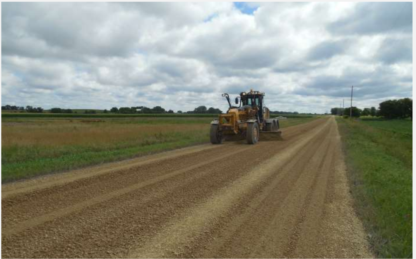
Grading new aggregate on 290th. Street.
