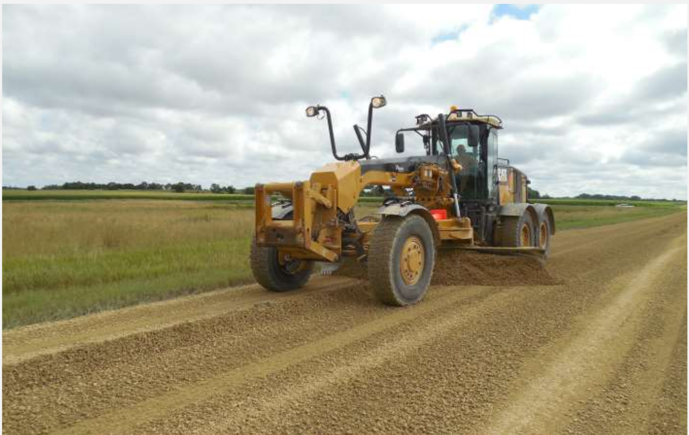
Grading new aggregate on 290th. Street.
