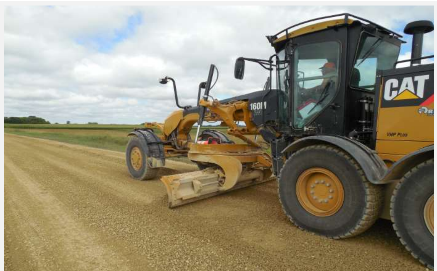
Grading new aggregate on 290th. Street.
