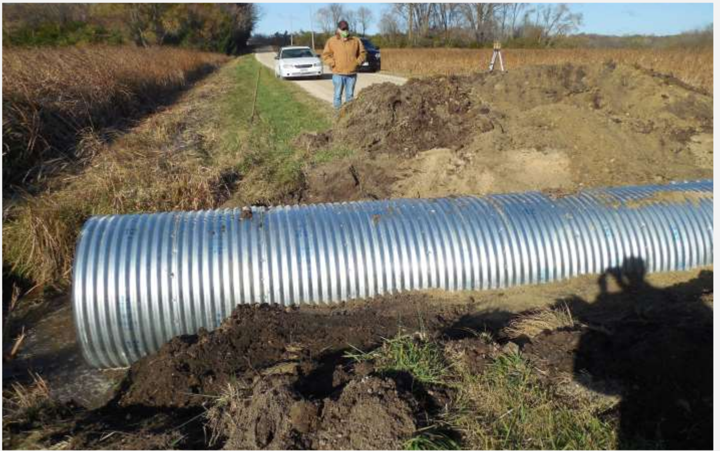
285th. Street culvert in place.
