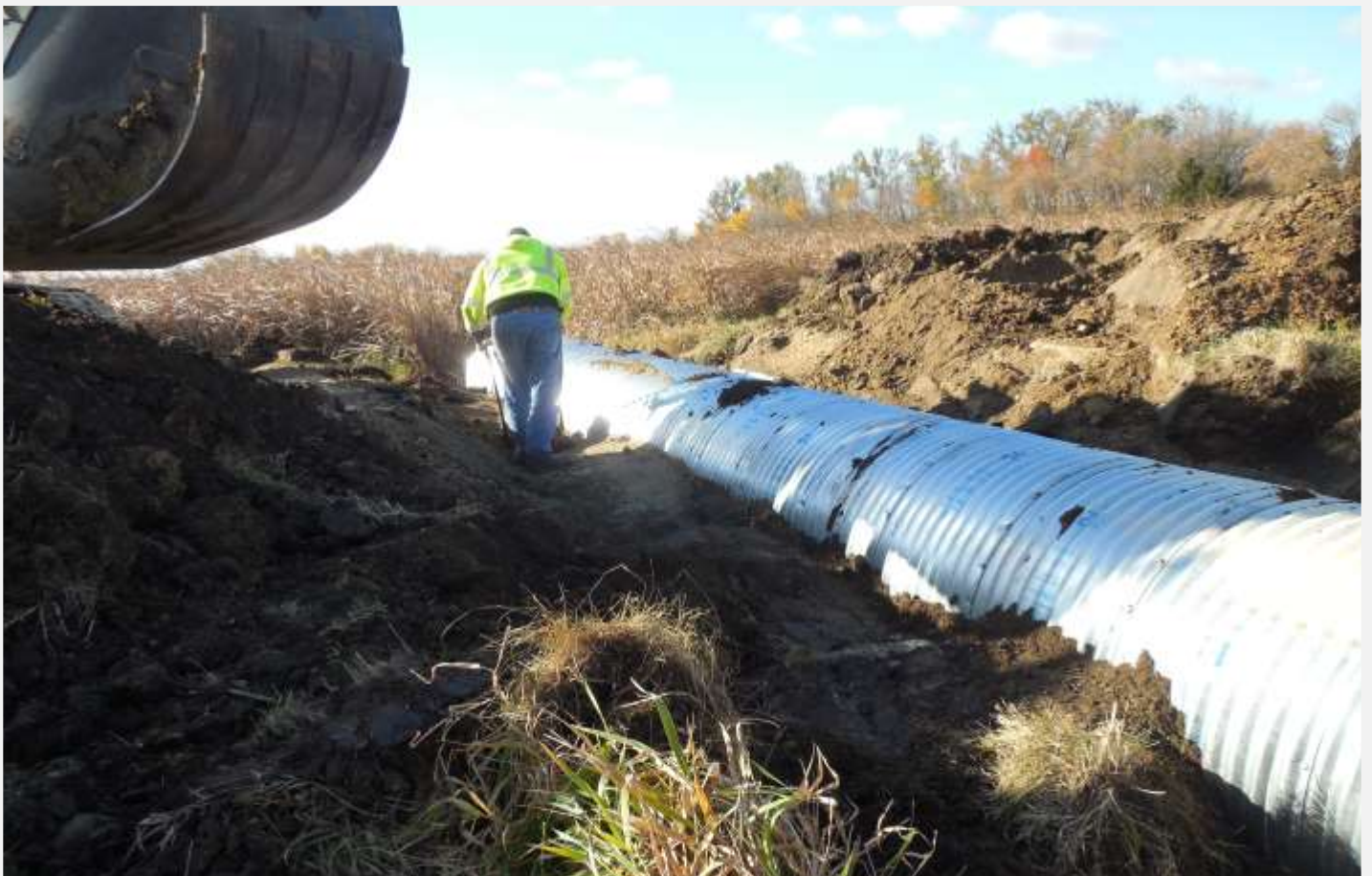
Placing the 285th. Street culvert.
