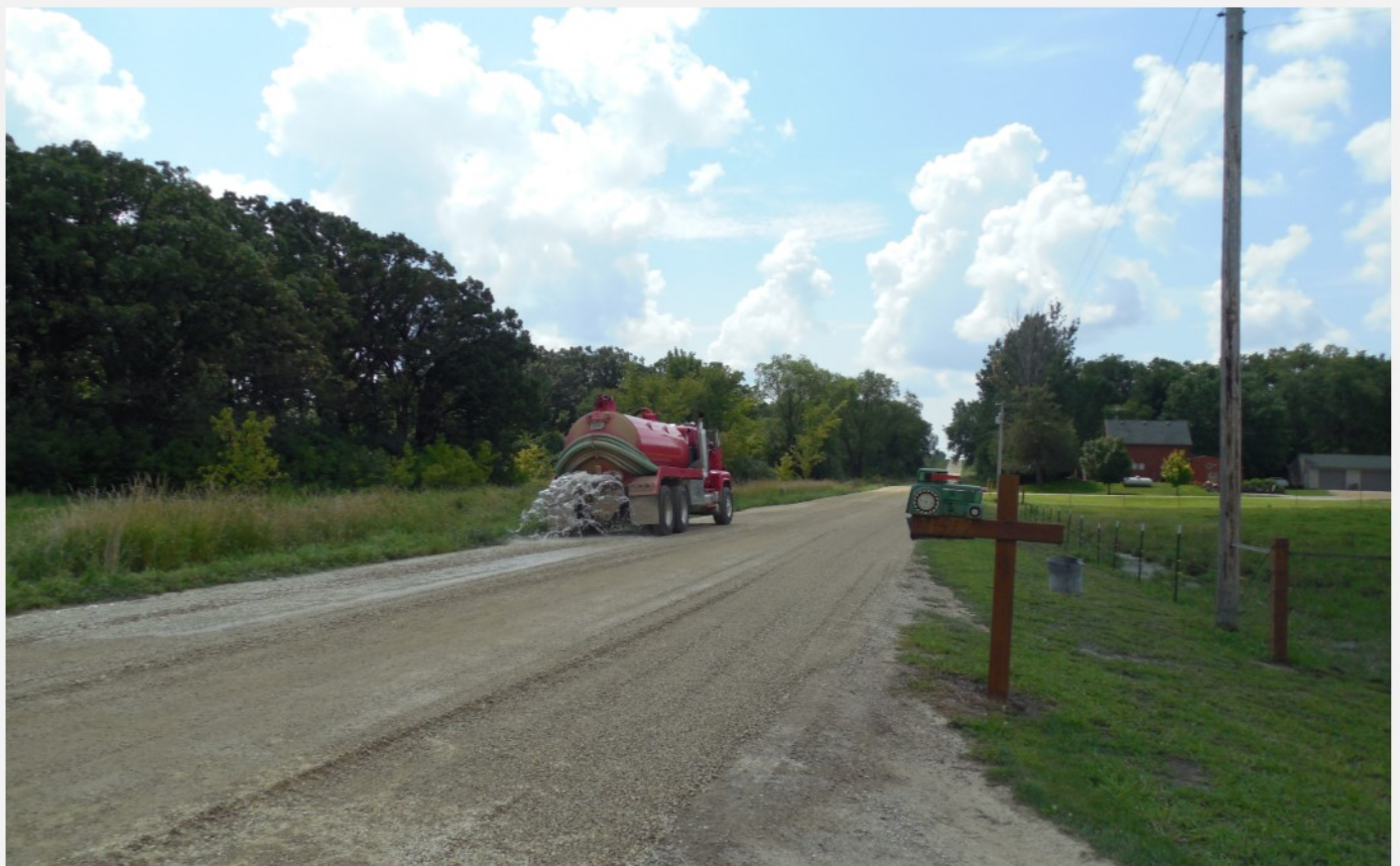
Watering Jamaica Avenue during grading work.
