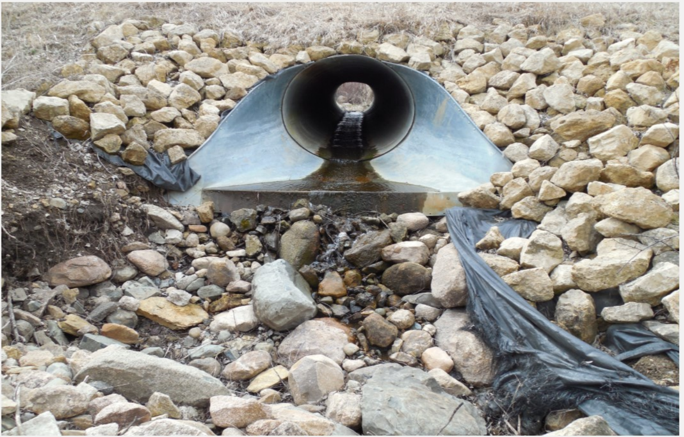
Washed out exit area of North Holyoke Avenue culvert before repairs.
