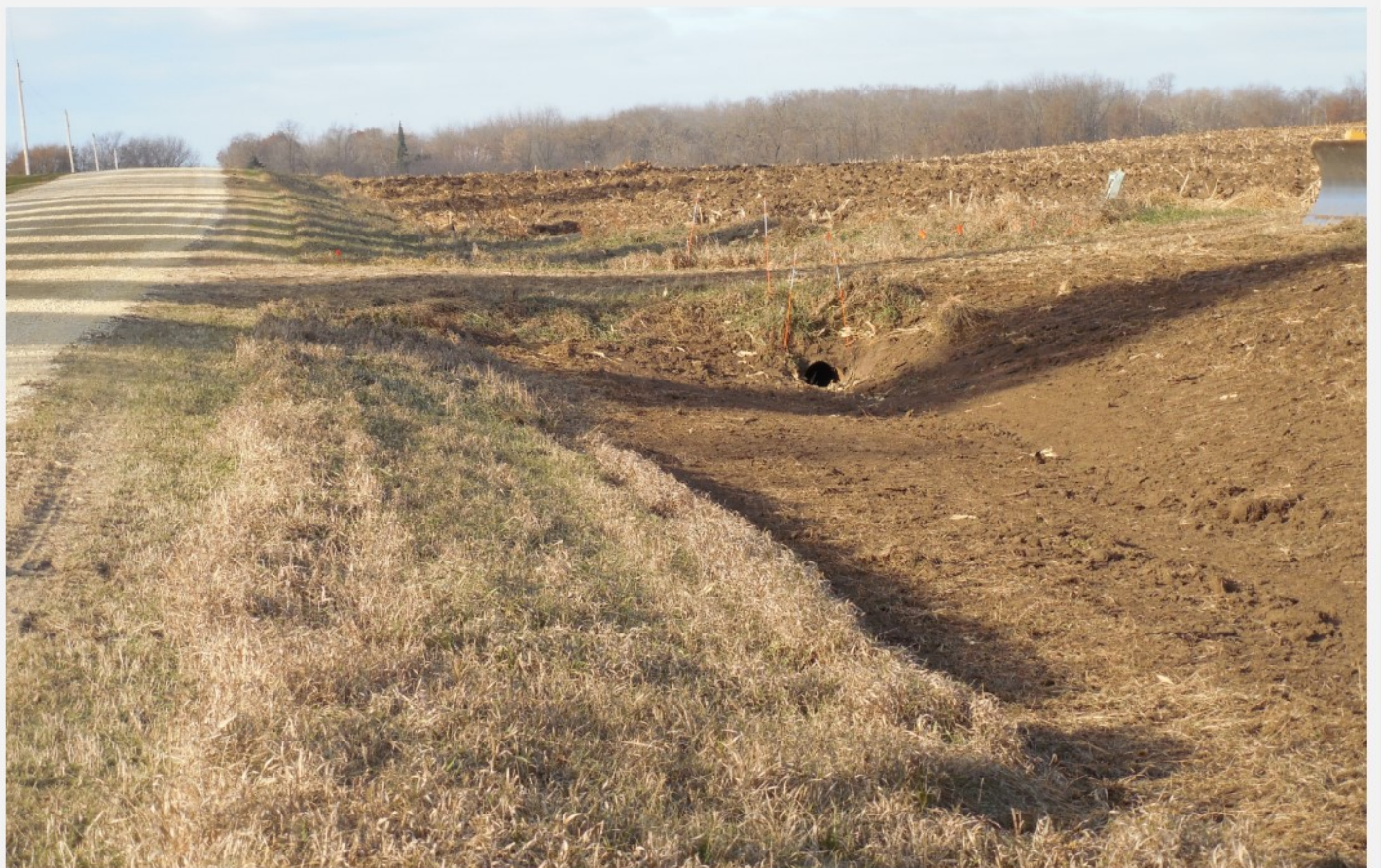
Ditch re-shaping in driveway areas on 300th. Street.
