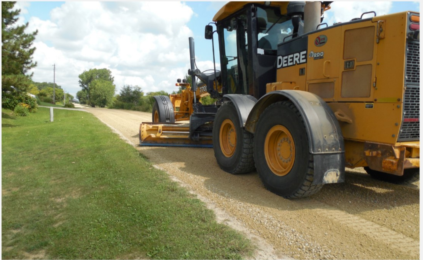
Finish grading the edge of Jamaica Avenue.
