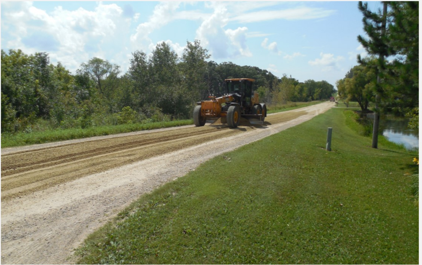
Grading Jamaica Avenue after new aggregate delivery.
