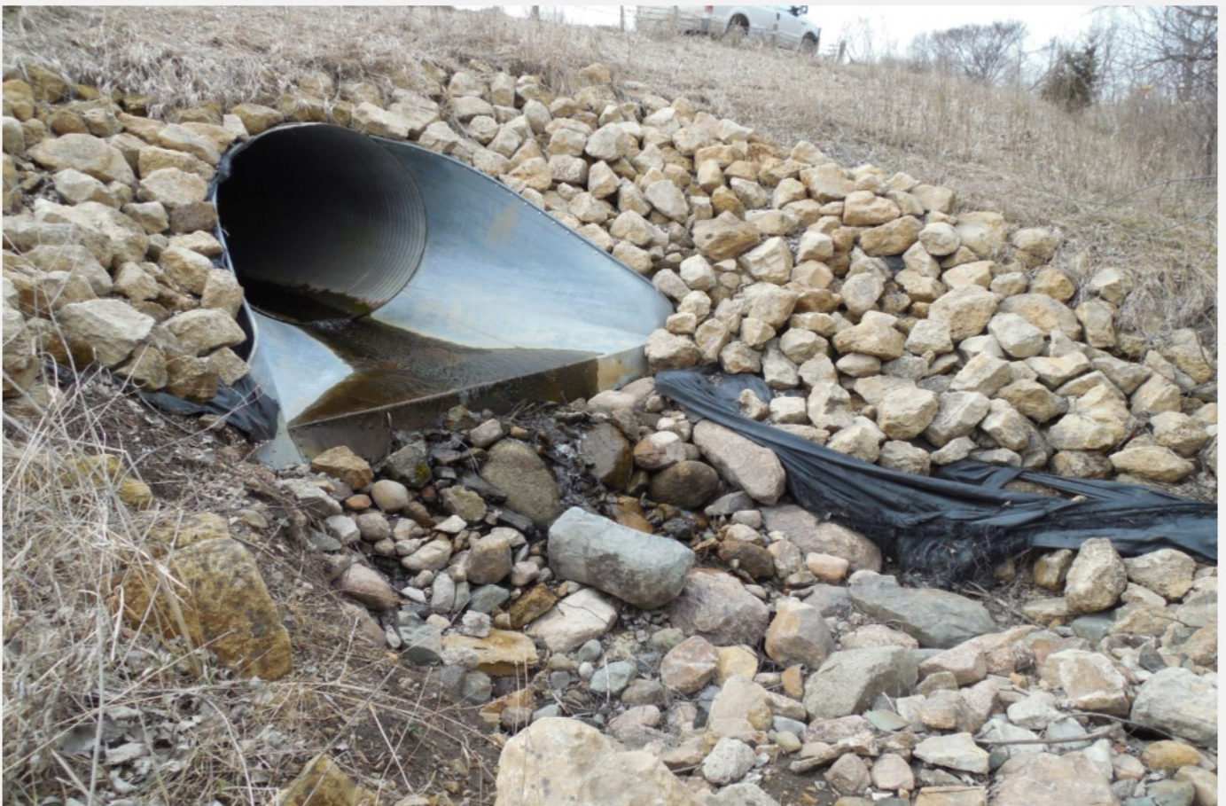
Lower exit area of North Holyoke Avenue culvert before repairs.
