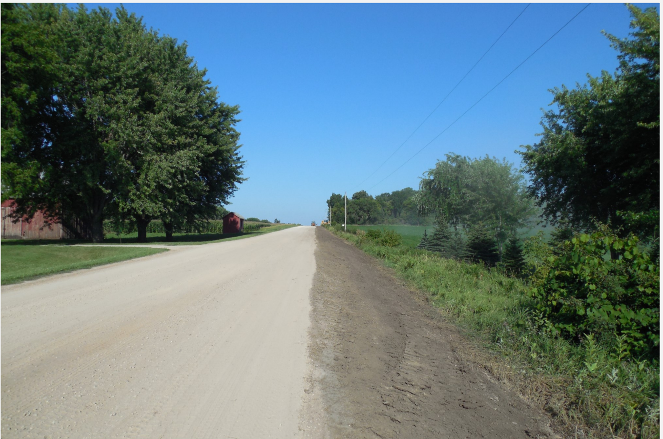
New aggregate surface on the west end of 315th Street
