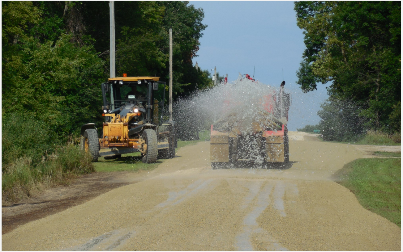
Watering and grading new aggregate on 315th Street
